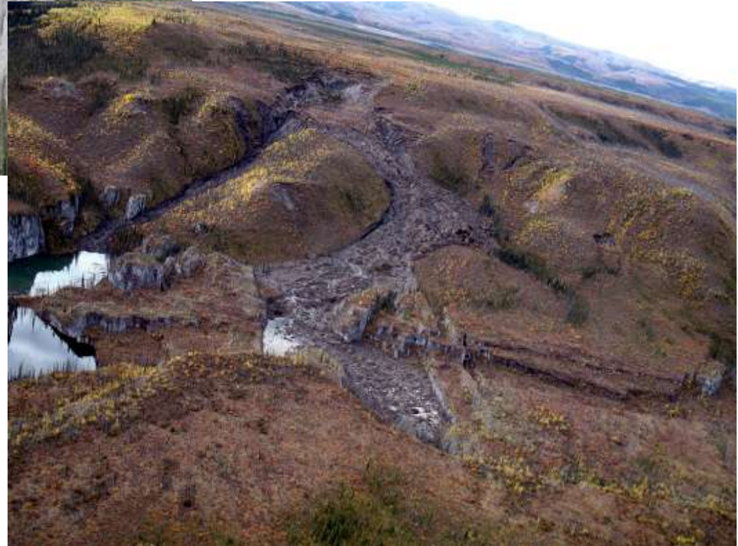
Right – the same scene in September 2009 after a landslide in glacial silts due to permafrost melting
